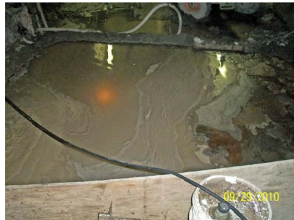
Figure 14. Another Photo Showing Precipitated Mud in the Sump
