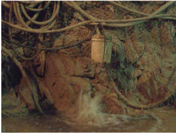
Figure 12. Z Clear 129 Injection Through Pump Tube
