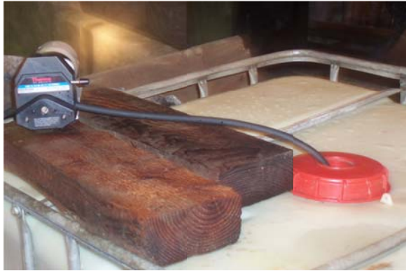
Figure 16. Polyamine Feed Pump from Tote
